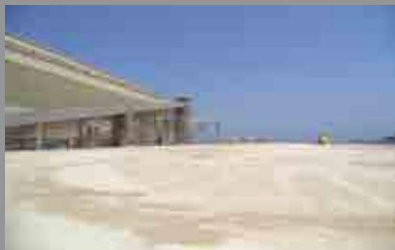
Old Silo area after demolition and reinstatement
