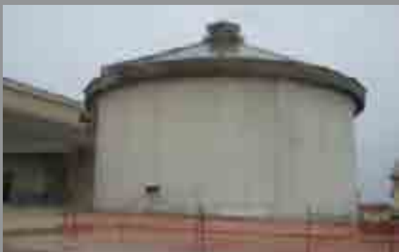
Old Silo before demolition
